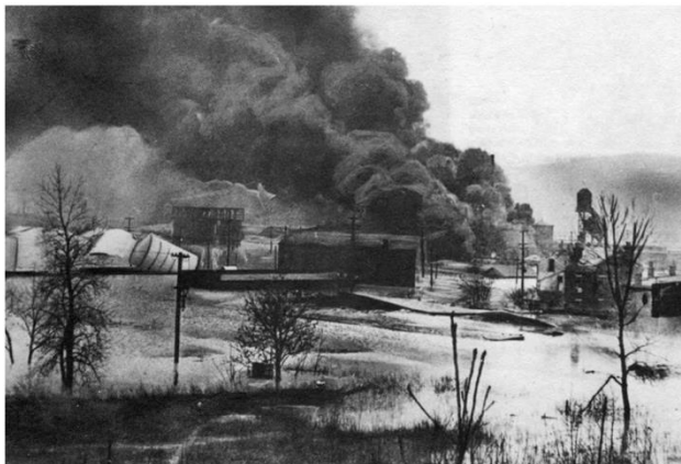
"Black Sunday" Gas tanks ruptured near Mill Creek that took firefighters over 12 hours to put out. Photo provided by Phil Lind
