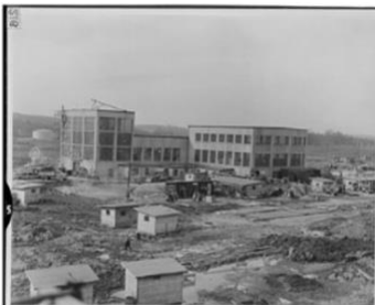
Pilot Plant under construction
